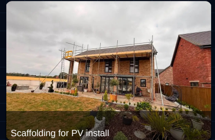
Scaffolding for PV install
